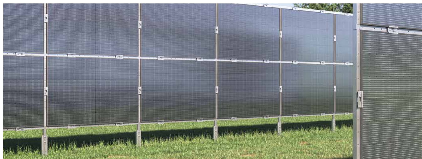
Agri-PV Vertical system
